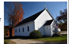
Former St. Joseph Church Before Renovation
