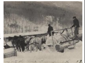
Snow Roller in Action— Livermore, NH 1921 (unfortunately, we don't have one of a Bartlett roller in action)
