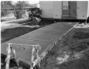
The new concrete sidewalk installed with a pitch to shed water to the road—just poured
