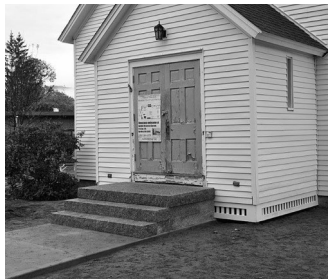
The new granite front steps at the entrance. Railings are yet to be installed. Base layer of grading is seen as is the new lattice work at the foyer's base
