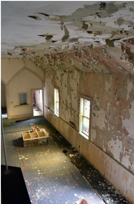
View of the south side wall and ceiling (right side of church) showing heavy water damage in the photo above and on the left; above photo shows area where plaster fell from ceiling; left shows peeling paint and deteriorating plaster.
