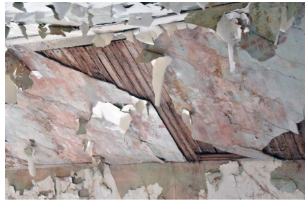
View of the south side wall and ceiling (right side of church) showing heavy water damage in the photo above and on the left; above photo shows area where plaster fell from ceiling; left shows peeling paint and deteriorating plaster.
