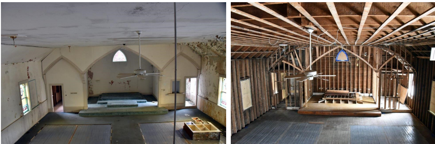
View of the front altar area from the choir loft, before demolition (l); after demolition (r)
