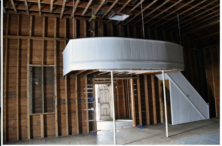
View of the church entry from the altar on the left and a slightly different angle on the right. We are planning to keep the choir loft in place. We needed to remove the confessional during the demolition. Notice the window frame that was covered in the wall in post demolition photo. There's an identical one frame behind the stairway to the choir loft. It's not known when they were covered.
