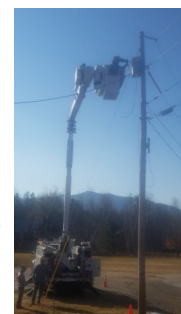
NH Electric Coop worker installs new service line
