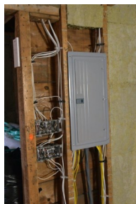
New electrical panel on the main floor level
