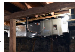
New 112,000 BTU Furnace hanging in basement
