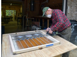
Worker sands off layers of paint
