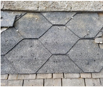
Above—Left first course of asphalt shingles found covering original wood shakes; Center & Right above, shows close-up shots of the south side roof deterioration. Most of this lower part of the roof was removed by hand and fell apart as it was touched
