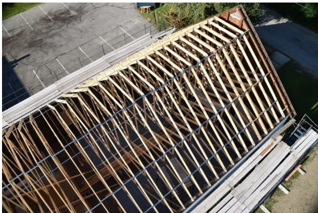
Roof Truss Installation
