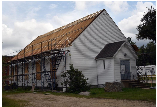
Roof Truss Installation
