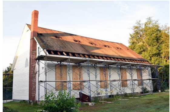
Above—Left, the south face of the building prepared for removal of the roof; Right is the north face of the building.
