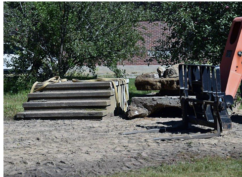
Concrete precast stairs set aside waiting to be disposed of; we know they were installed prior to 1955 based on dated photographs but we don't have an exact installation date; the original steps for the church were wooden
