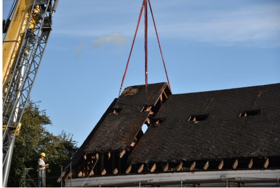
The first section of the building is lifted off the building and airborne
