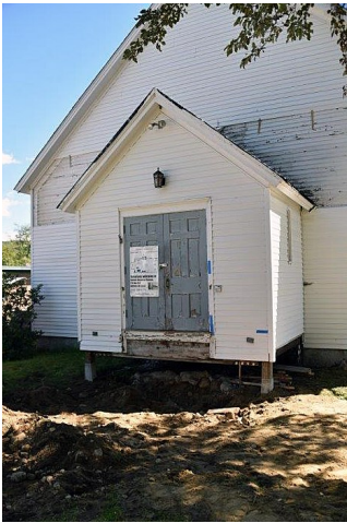
View of the front of the building, foyer level, stairs and walkway removed
