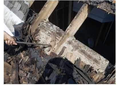
Above—Left first course of asphalt shingles found covering original wood shakes; Center & Right above, shows close-up shots of the south side roof deterioration. Most of this lower part of the roof was removed by hand and fell apart as it was touched
