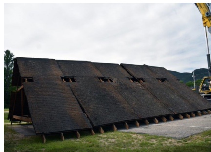
More roof sections are removed from the building
