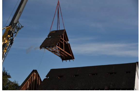
The first section of the building is lifted off the building and airborne
