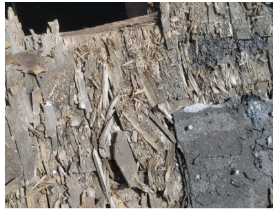
Above—Left first course of asphalt shingles found covering original wood shakes; Center & Right above, shows close-up shots of the south side roof deterioration. Most of this lower part of the roof was removed by hand and fell apart as it was touched
